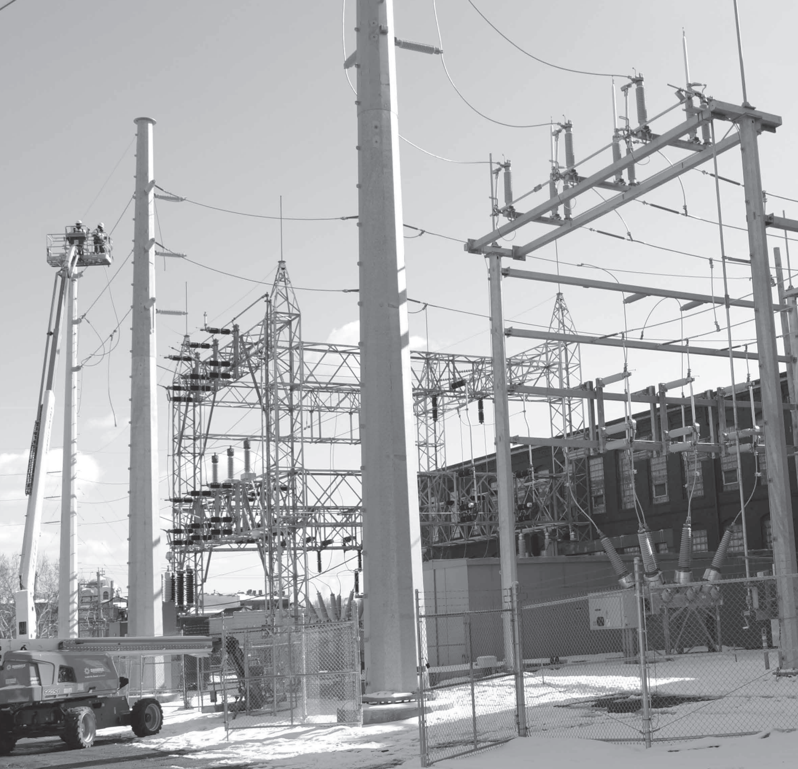
17L Substation Project
