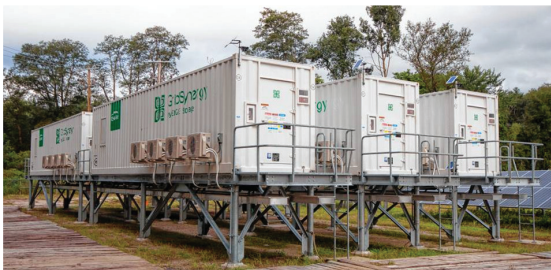
Energy Storage Systems (ESS) are used to enhance HG&E's electricity system and help keep electric rates stable by reducing rising demand charges for the utility and its customers.
