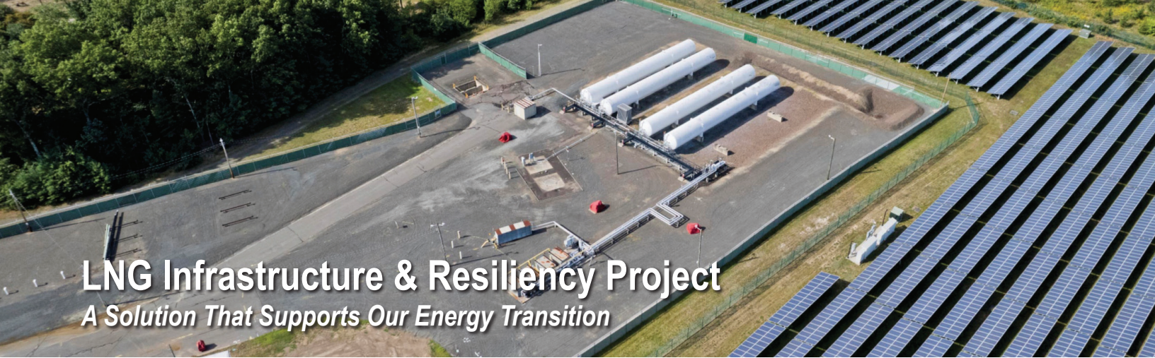
West Holyoke LNG Facility current footprint, four tanks with a foundation for a fifth tank.
